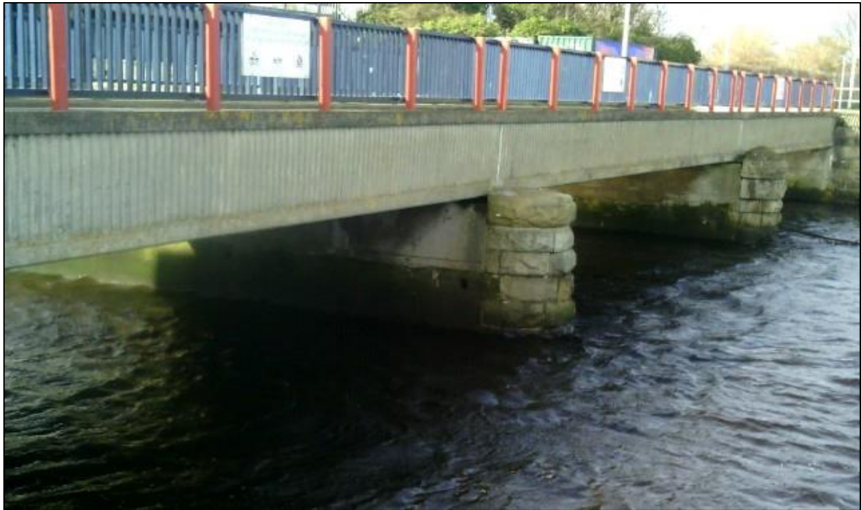
Figure 15 - Road Bridge at Section 16 Looking Upstream
